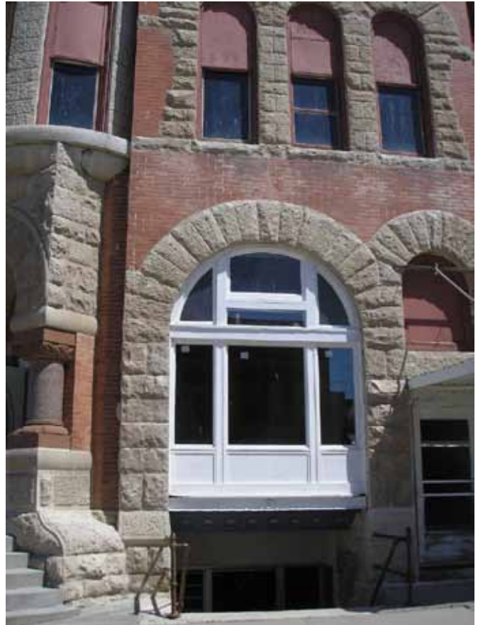
Repaired arched front window, First National Bank building (2009)
